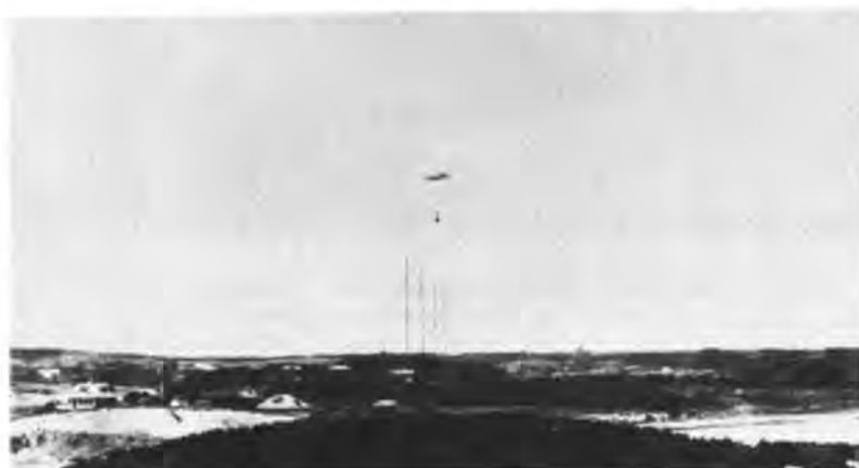
1919 - June 13th. The Marconi Receiving Site North Chatham, Mass. 350 Ft. Masts Supporting Beverage Long Wave Antenna System.
